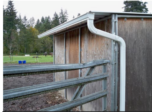
A roof runoff structure like the one seen in the picture helps to collect, control, and transport precipitation from roofs. Picture courtesy of the King Conservation District.
